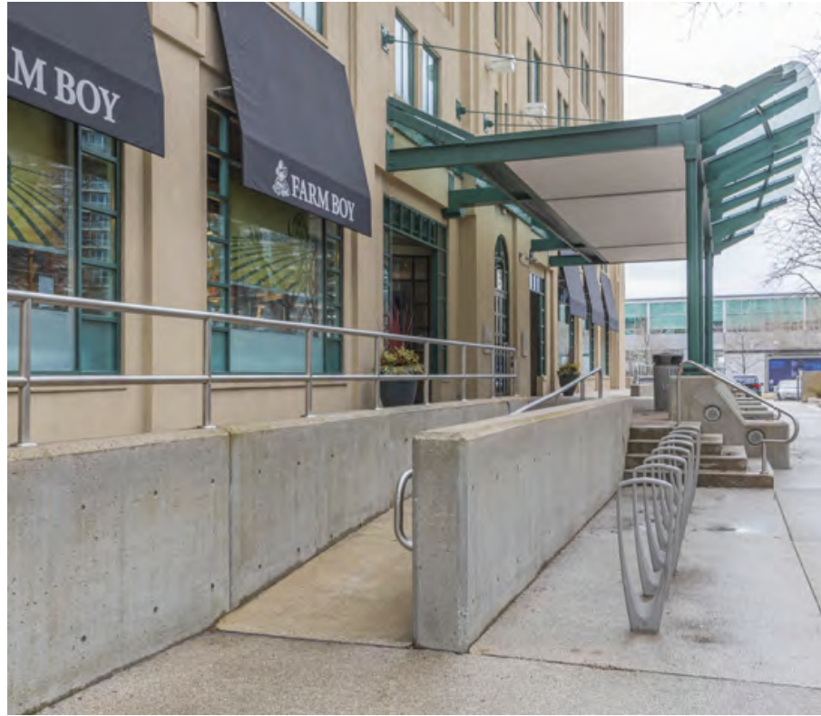
Image Description: The doors to the Queen's Quay Terminal building (north east entrance).
