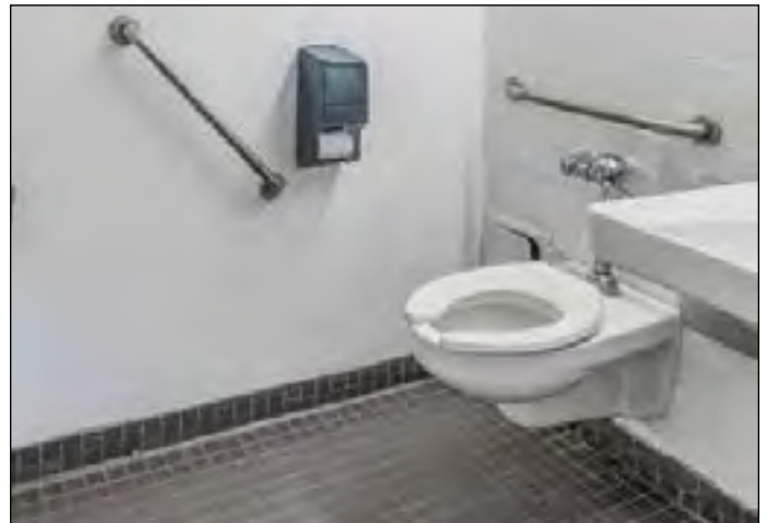
This is an image of inside the restroom on the main floor.
