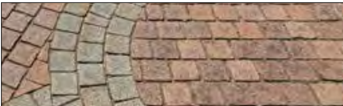
This is a photo showing the brick ground covering.
