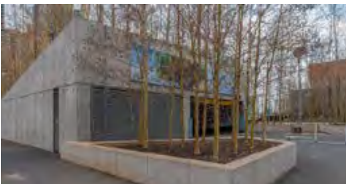
This is an image of the entrance to the parking garage at 235 Queens Quay West.
