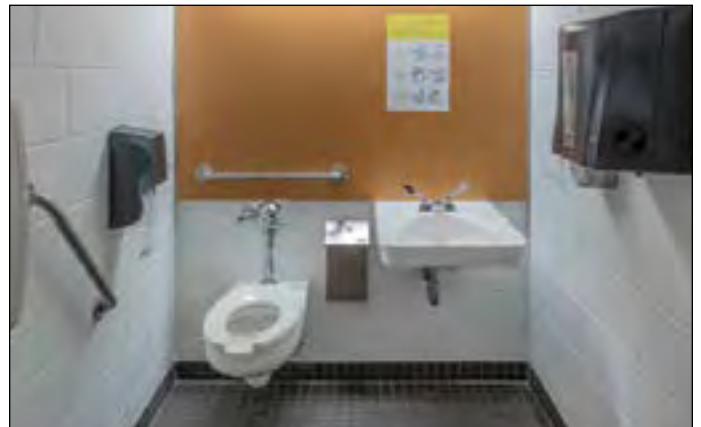
This is an image of inside the upper lobby restroom.
