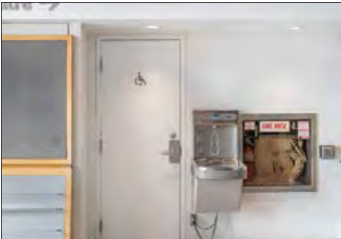
This is an image of the door of the accessible restroom on the main floor of the building.
